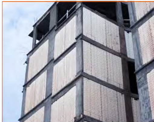
PANEL INSTALLED IN CONCRETE FRAME STRUCTURE
