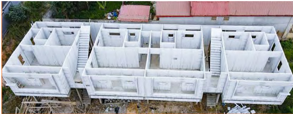
INSTALLED PANEL
